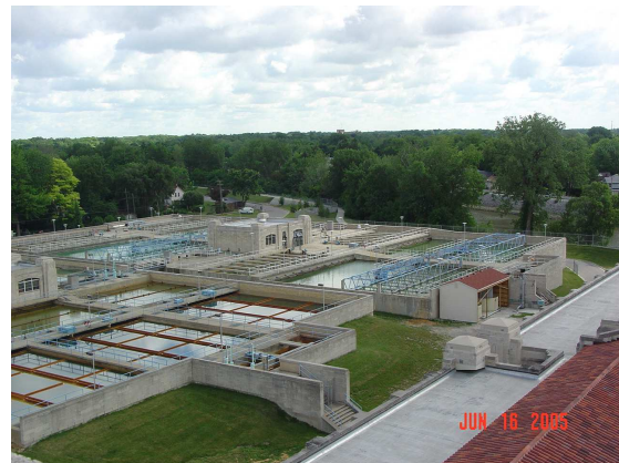
Settling basins on the south side of the Plant
