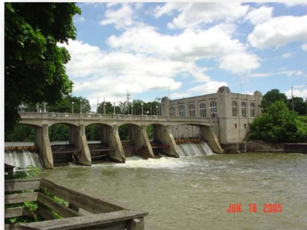
St. Joseph River Dam
