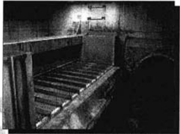
ACU-SCREEN in stormwater overflow basin.
