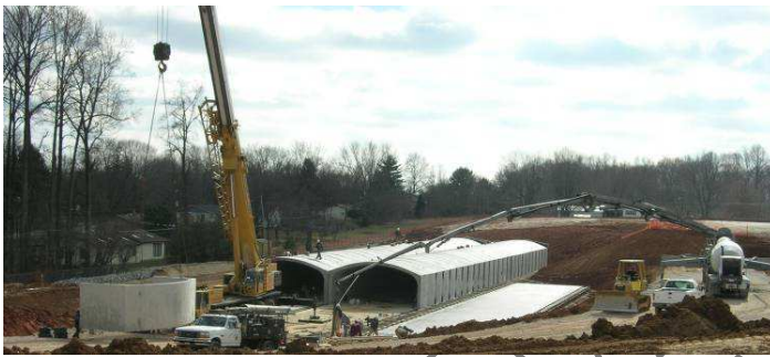
CONTECH® SUBSURFACE VAULT – KMART, BLOOMINGTON, IN
