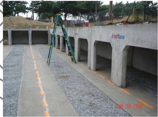
STORMTRAP® SUBSURFACE VAULT WITH INFILTRATION, GARY, IN
