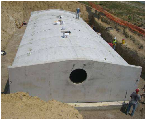
CONTECH® SUBSURFACE VAULT, FEDERAL EXPRESS® FACILITY – INDIANAPOLIS AIRPORT
