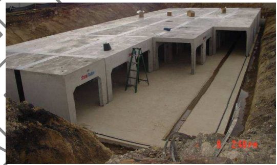
STORMTRAP® SUBSURFACE VAULT - MUNICIPAL BUILDING, LEBANON, IN
