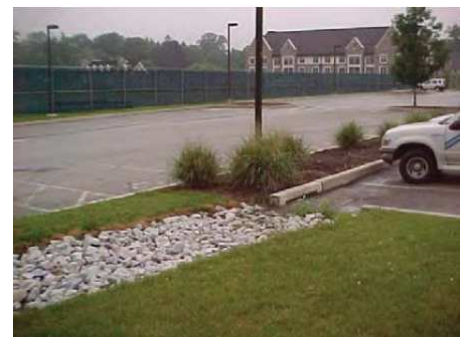
FILTER STRIP PROVIDING PRETREATMENT FROM A PARKING LOT TO A BIORETENTION SYSTEM
