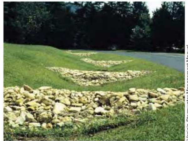
CHECK DAMS: NOTE CHANNEL STORAGE CAPACITY CREATED BY CHECK DAMS. NOTCHED CENTER ALLOWS SAFE OVERFLOW WITHOUT SCOUR AROUND SIDES
