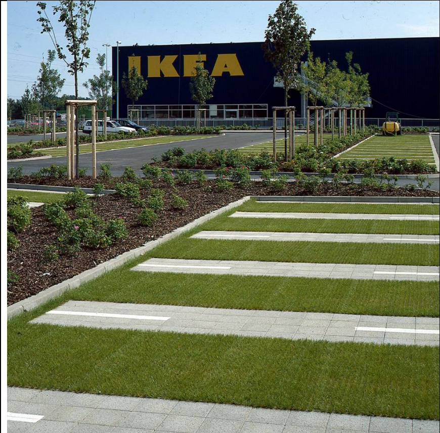
IKEA Parking Lot ◆ Permeable Pavement ◆ Bioretention
