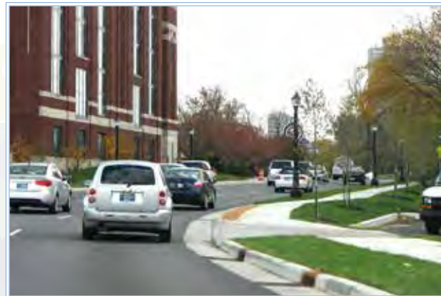
Recent improvements to Clinton just south of State Boulevard will soon be extended to Fourth Street.
