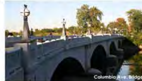
Columbia Ave. Bridge
