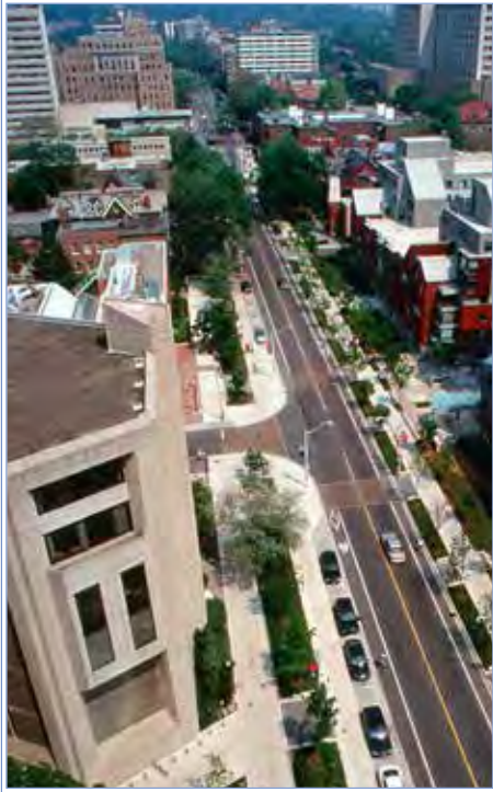
Context Sensitive Solutions (CSS) considers a roadway's surrounding context and land use needs, as seen here with this urban roadway in Toronto, which has been reduced in width to accommodate pedestrians, bicyclists, and parking needs.
