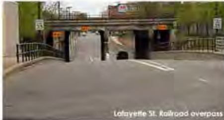
Lafayette St. Railroad overpass
