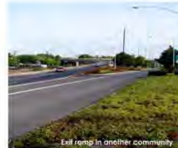
Exit ramp in another community
