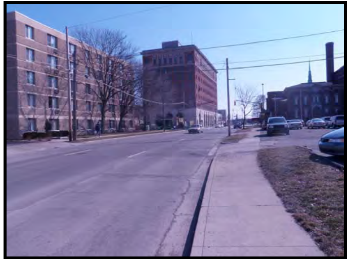
Facing south at Ewing St. and Main St. Intersection
