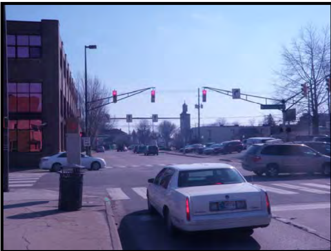
Facing south at Fairfield Ave. and Washington Blvd. Intersection
