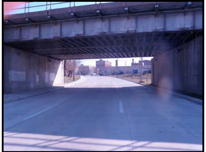
Facing south on Ewing St. at Railroad Underpass
